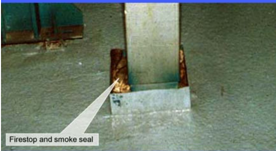
Electrical and other service shafts :
