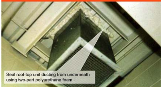
Roof-mounted HVAC equipment:
